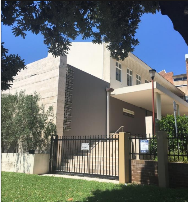
Picture 1 – Shule Building and Pedestrian Access from Napier Street
